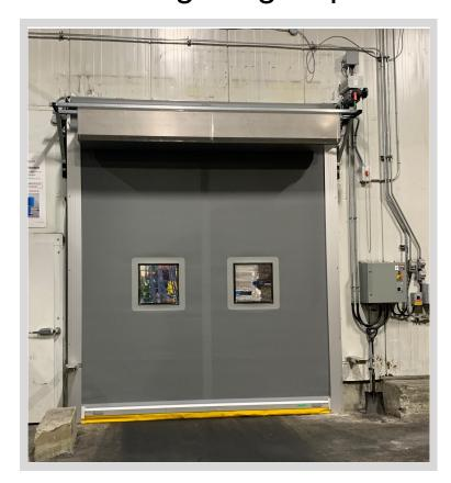
NEMA 4-12 Control panel with multi-tap transformer compatible with 208v-240v, 460v-480v and 575v-600v in single phase
